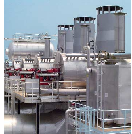
Four RGL70 burners on thermal fluid boilers ensure the crude oil can be pumped
